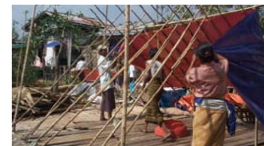
Above: Temporary housing is erected in Burma
